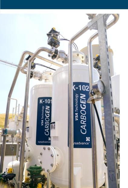
**CARBOGEN** is a cleantech VPSA for capture and purification of CO2 from:
