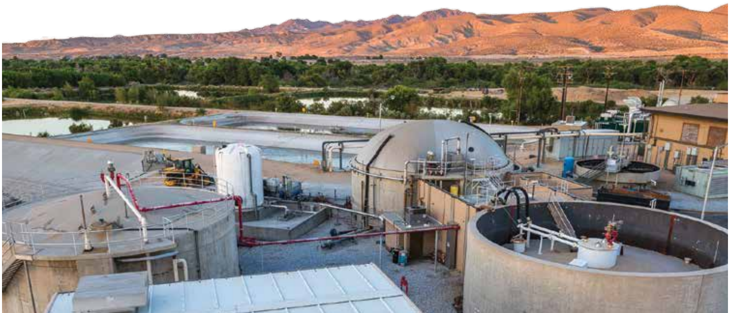
An anaerobic digester at the Victor Valley Wastewater Reclamation Authority (VWRA) in Victorville, California converting organic waste and sludge into renewable energy using Anaergia’s Omnivore™ high throughput anaerobic digestion technology.
