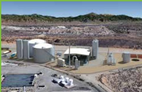
Rialto Bioenergy Facility (Rialto, CA)
