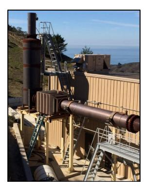
Figure 17. View of Exhaust System of the One Unit (this unit previously included both oxidation and SCR catalysts)
