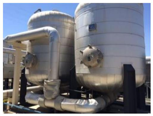
Figure 23. General Setup of Vessels for the Siloxane Removal System (Four vessels are incorporated into the system)
