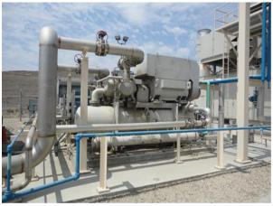
Figure 27. Gas Compressors Arrangement
