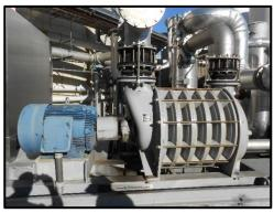
Figure.13. Biogas Compressor at East Bay MUD
