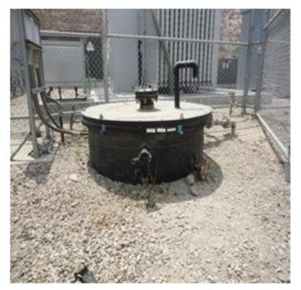
Figure 26. V-120 Condensate Holding Tank
